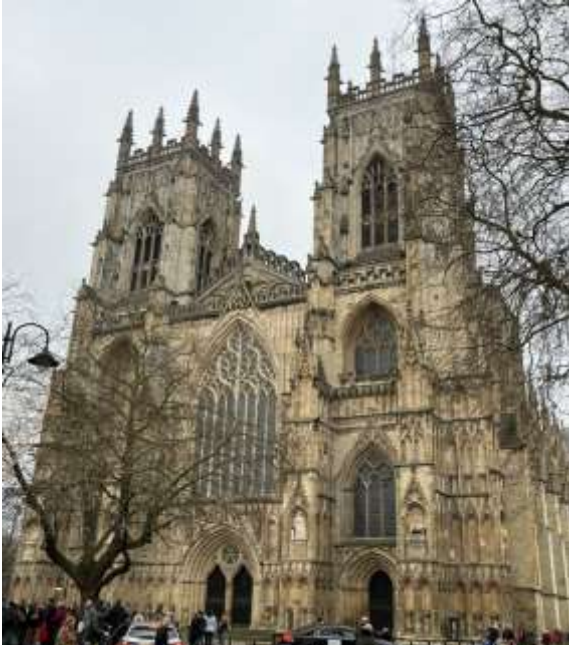
West façade, and entrance, York Minster
